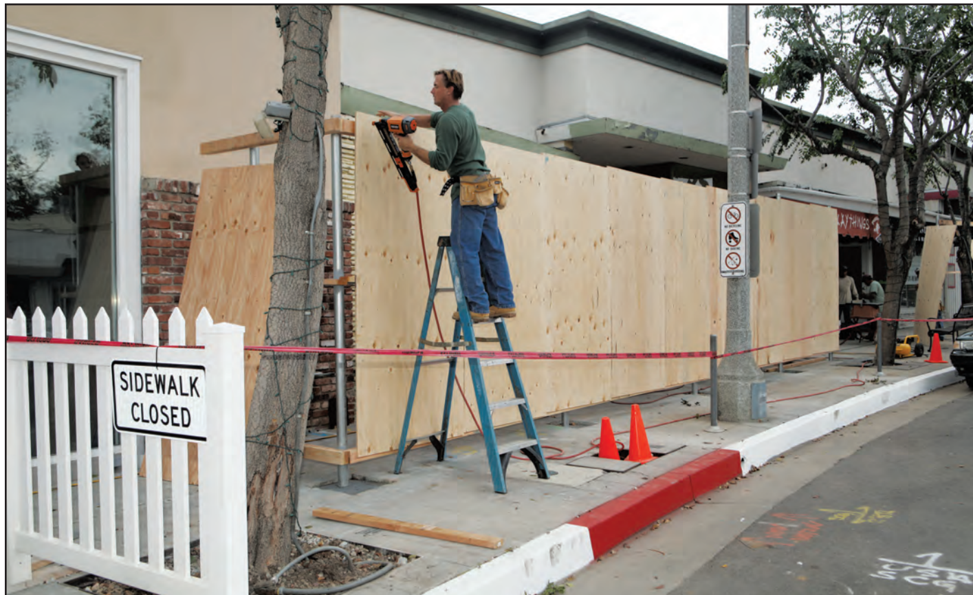
A construction fence has gone up around the buildings on the north side of Swarthmore before demolition begins. Photo: Bart Bartholomew
