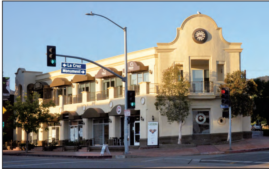
The Clock Tower Building has a new owner, who may make upgrades. Photo: Shelby Pascoe
