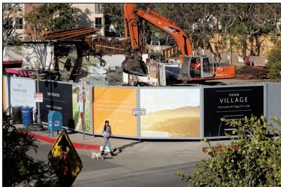
Village Books was located where the crane operator is at work.
