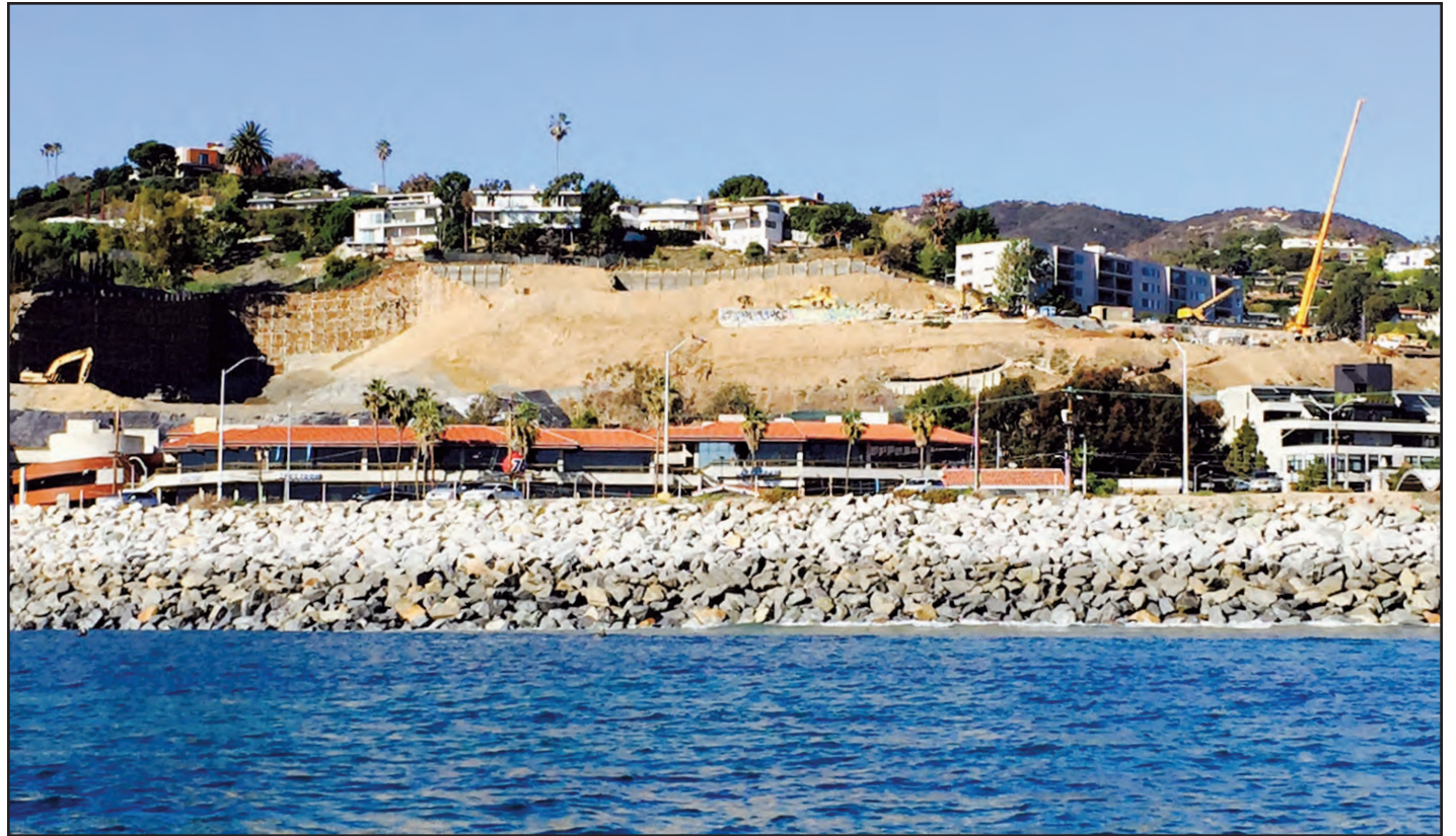
Eighty-two units will be built on the Revello landslide in the lower Castellammare area. Excavation is underway. Photo: Reece Pascoe
