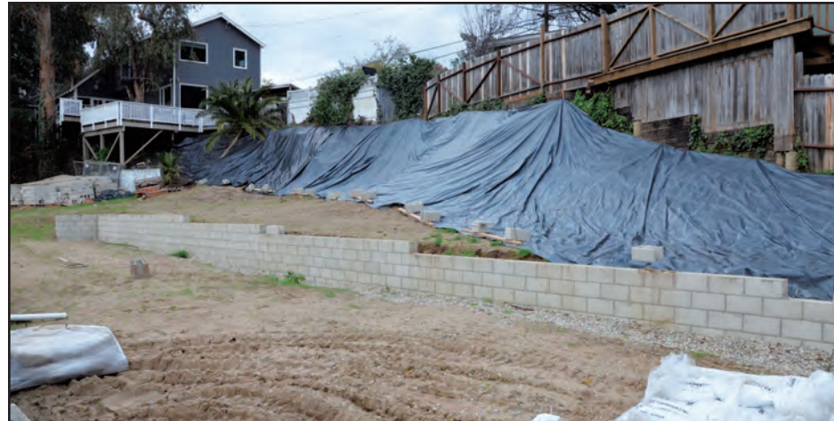
The proposed nursery at 810 Temescal Canyon Road, across from the high school, is on hold pending a grading permit.
