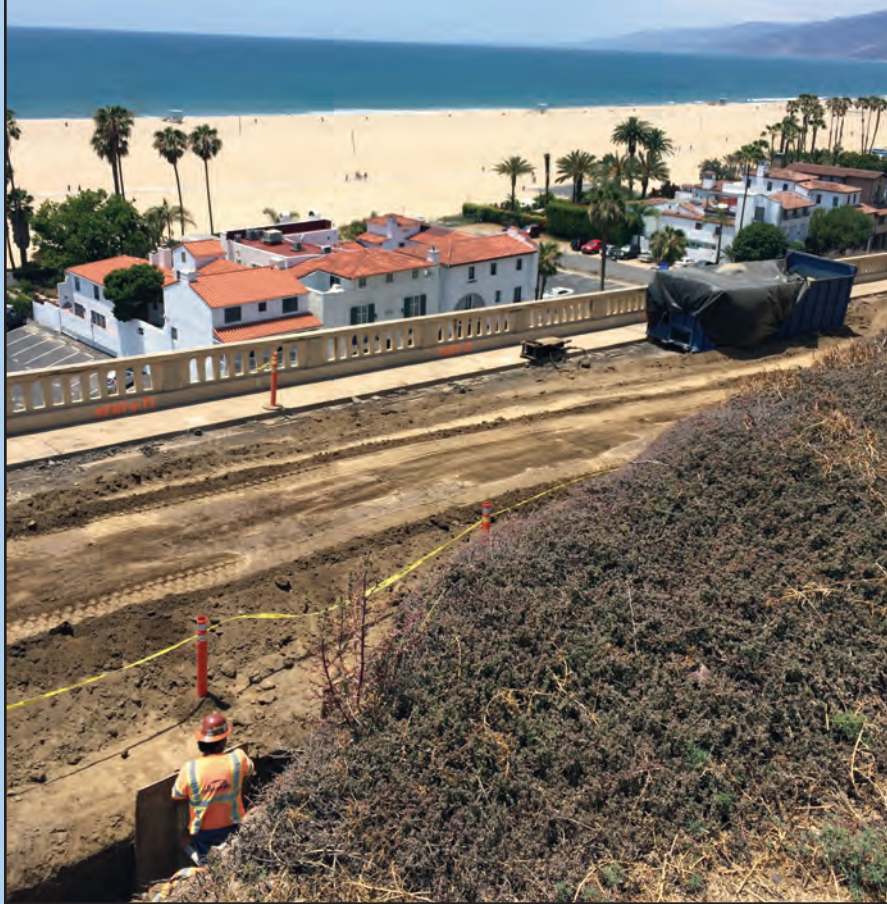
The California Incline in Santa Monica finally closed April 20, six years after the 1930s-built bridge was deemed seismically unsafe. The Incline replacement construction is scheduled for completion by May 2016. Photo: Wendy Anderson
