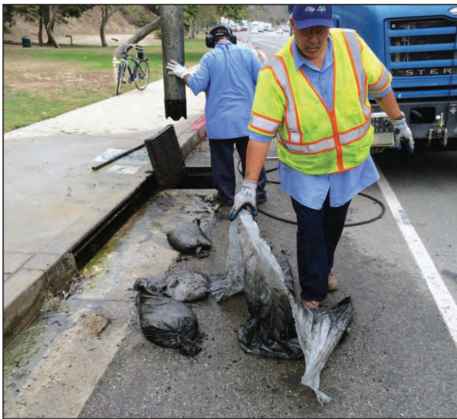
Sand bags were discovered plugging the storm drain, which remains partially blocked despite vacuuming efforts by City sanitation workers.
