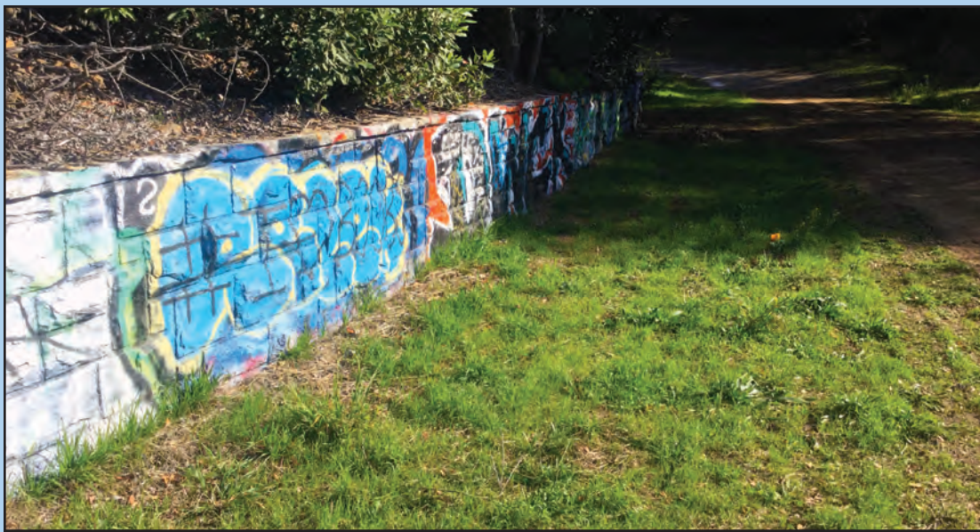
This wall at Murphy Ranch will remain, but hopefully the graffiti will be removed in this L.A. City park.
