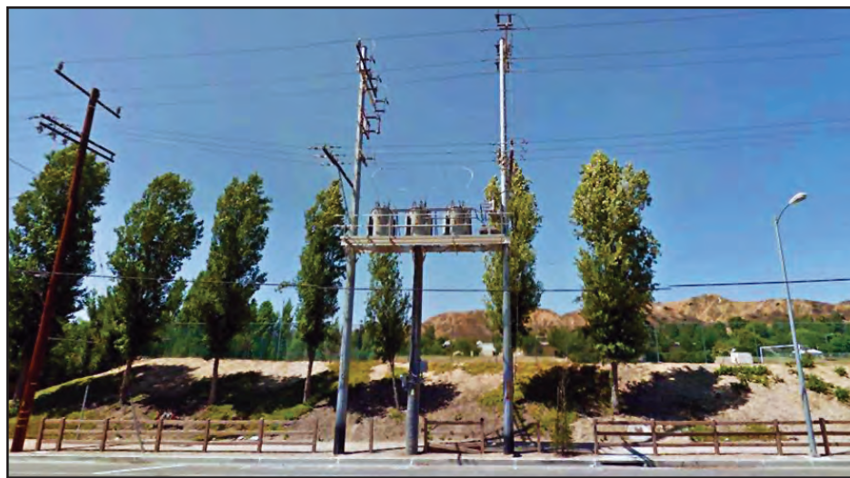
DWP pole-top stations will be installed at Marquez Ave. and El Medio Ave.
